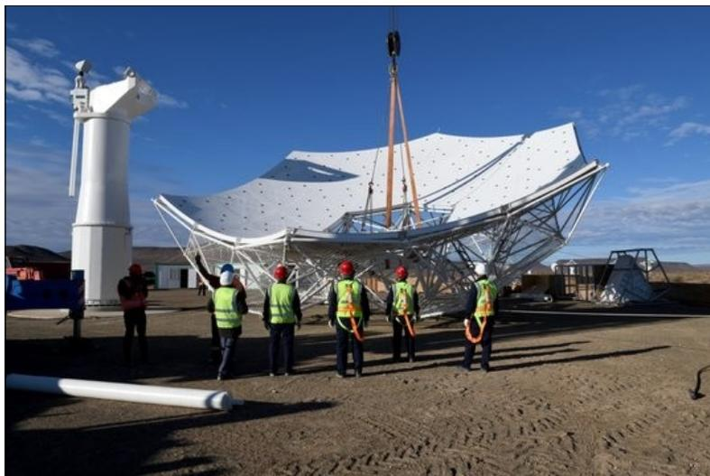
Reflector of the SKA-MPG Telescope of 15 m diameter just before mounting (Karoo Desert, South Africa).
