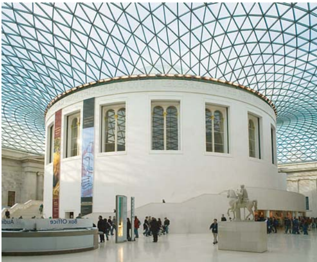
Fig. 1 British Museum Great Court Roof, London, UK (Courtesy of Andrew Dunn)
