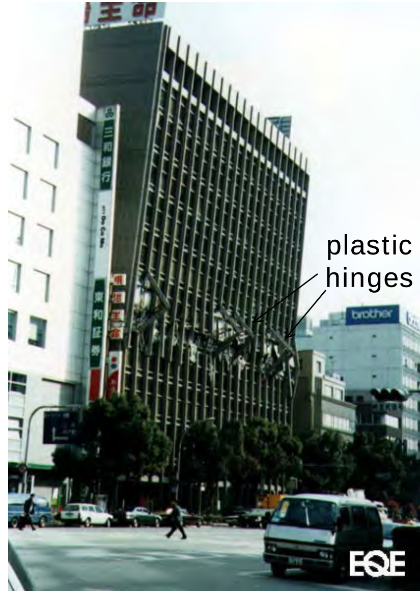
Mid-story collapse, 1995 Kobe earthquake (EQE Summary Rep., 1995)
