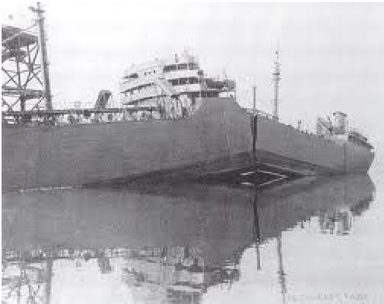
Liberty ship split in half on reaching the ductile-to-brittle transition temperature (Photograph courtesy of the Principle and Fellows of Newnham College, Cambridge)
