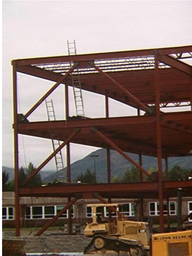
Figure 6.19. Example of a braced steel-frame.
