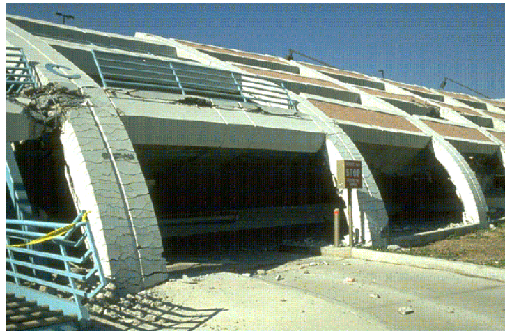
Figure 6.17. Example of ductile deformation of concrete columns from the 1994 Northridge earthquake. Adequate spiral reinforcing resulted in more ductile behavior than was shown in Figure 6.14.
