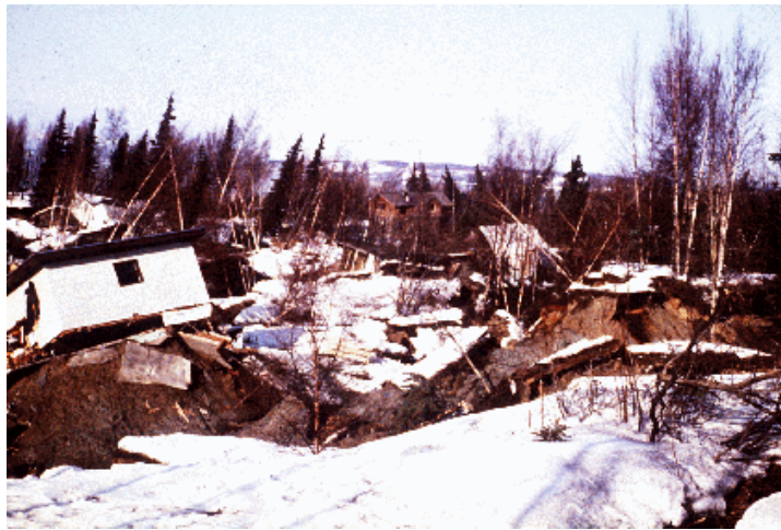
Figure 6.22. Wood frame houses that rode through the massive landslide triggered by the 1964 Alaskan earthquake.
