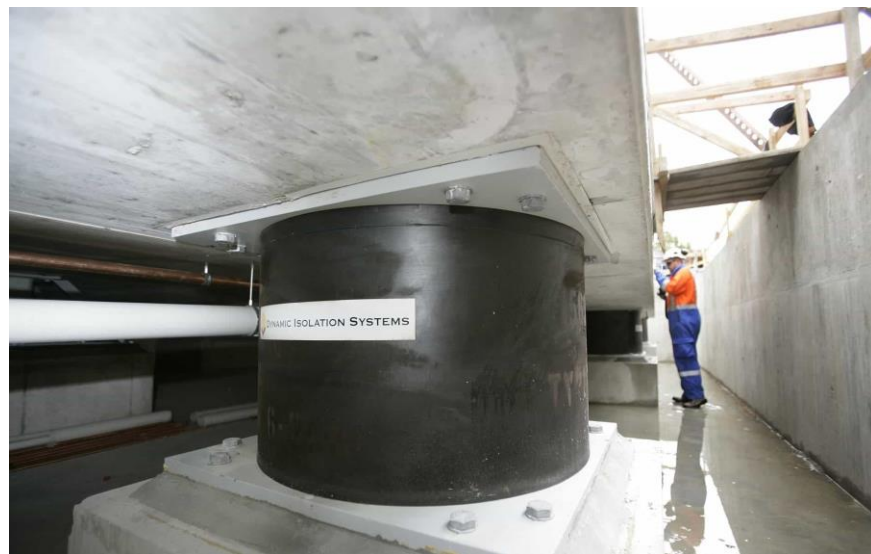
Figure 6-22. Base Isolated structure. The large black cylinder is one of many rubber/steel plate composite isolators that supports the weight of the building. The isolators are stiff in compression and flexible in shear. The concrete wall behind the engineer is the safety stop. The ground floor of the building is a massive reinforced concrete element that ensure that the ground floor moves as a rigid block.
