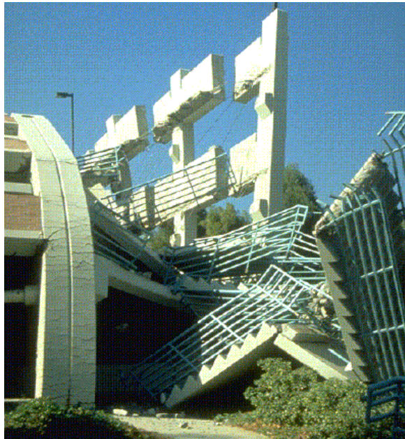
Figure 6.18. Despite the ductile behavior of the concrete columns, this parking structure collapsed because the floor slabs were not adequately connected to the rest of the structure. That is, the beams and columns were ductile, but the connections between these elements were not.
