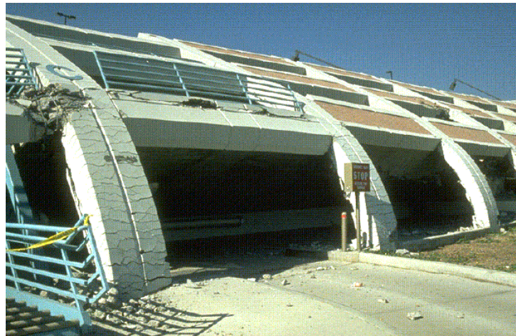
Figure 6.17. Example of ductile deformation of concrete columns from the 1994 Northridge earthquake. Adequate spiral reinforcing resulted in more ductile behavior than was shown in Figure 6.14.
