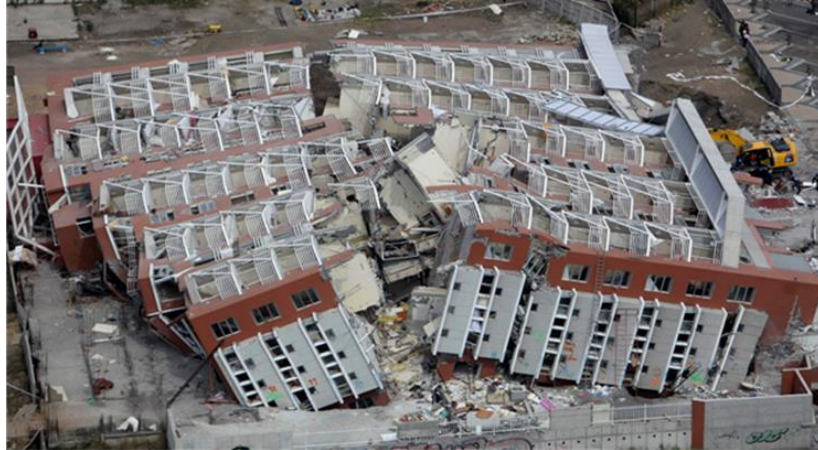
Figure 6.79. Collapse of a shear wall building in the 2010 Maule earthquake. Notice that although the building collapsed, the high strength of the shear walls preserved the integrity of most of the interior rooms. Fortunately, the area on which the collapsed building landed was unoccupied.
