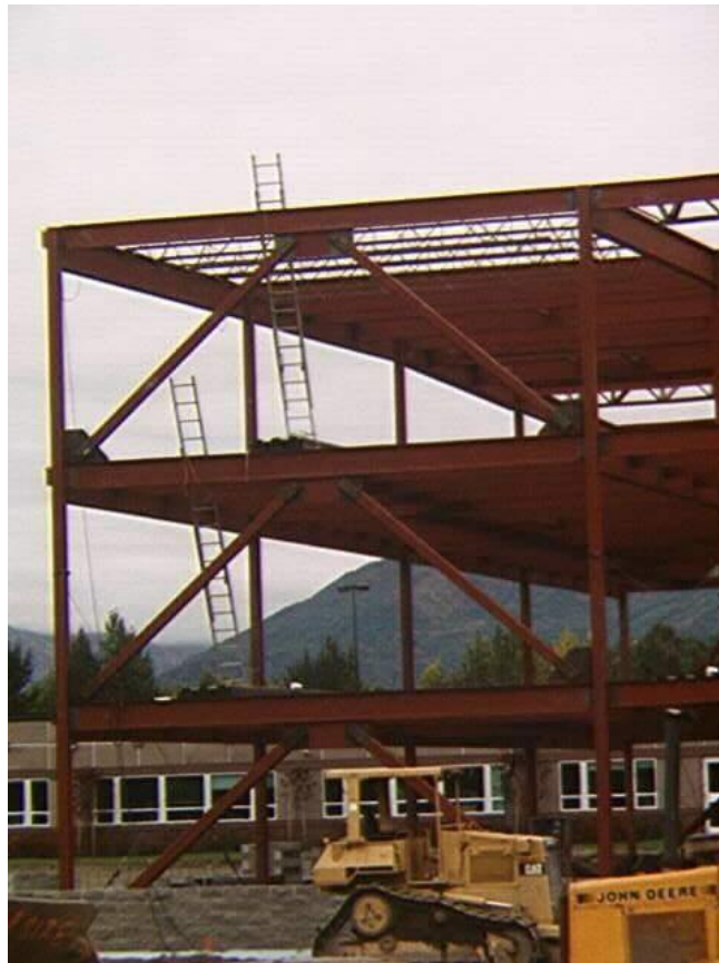
Figure 6.19. Example of a braced steel-frame.
