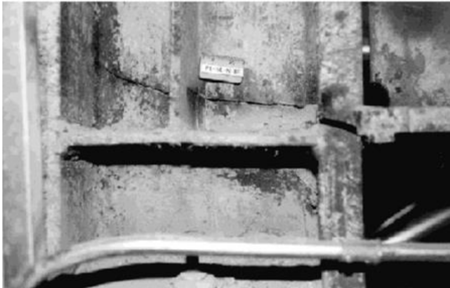
Figure 6.8. Example of a welded steel connection that fractured in the 1994 Northridge Earthquake. Notice that the weld between the flanges experienced a tensile crack that extended across the web of the steel column. Prior to this earthquake, it was generally believe that mild structural steel would ductily bend, but that it would never fracture. .
