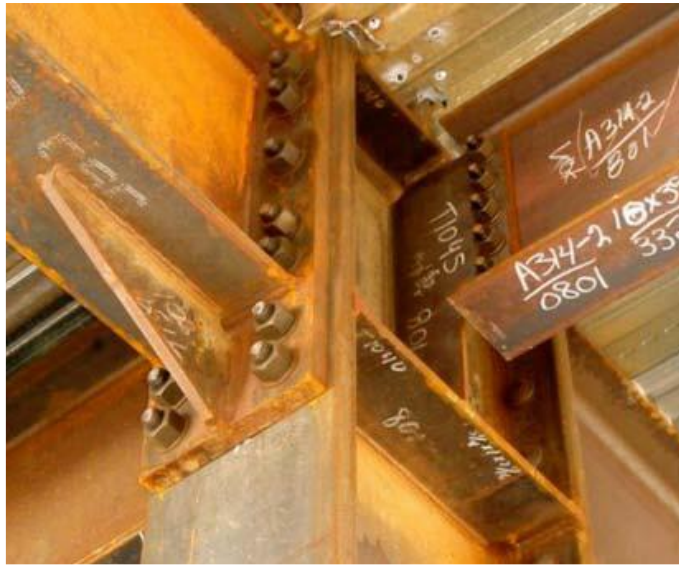
Figure 6.9. Post Northridge Special Moment Resisting connection (welded and bolted) in one direction and simple connection in the orthogonal direction
