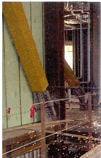
Unbonded Brace in the Broad Center
